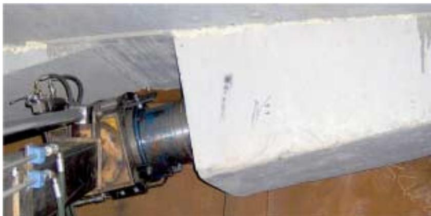
Fig. 3 Prestressing duct inside the box girder deck.
