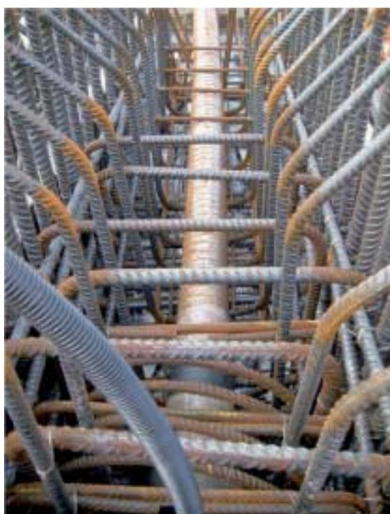
Fig. 4 Reinforcement alongside the duct.
